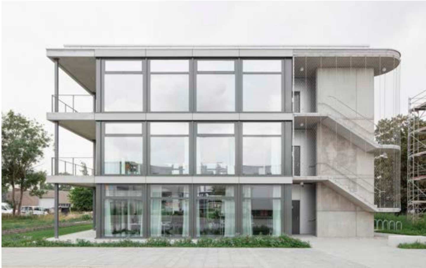
Figure 2.1. Exterior elevation of the TINA office-to-residential conversion.
