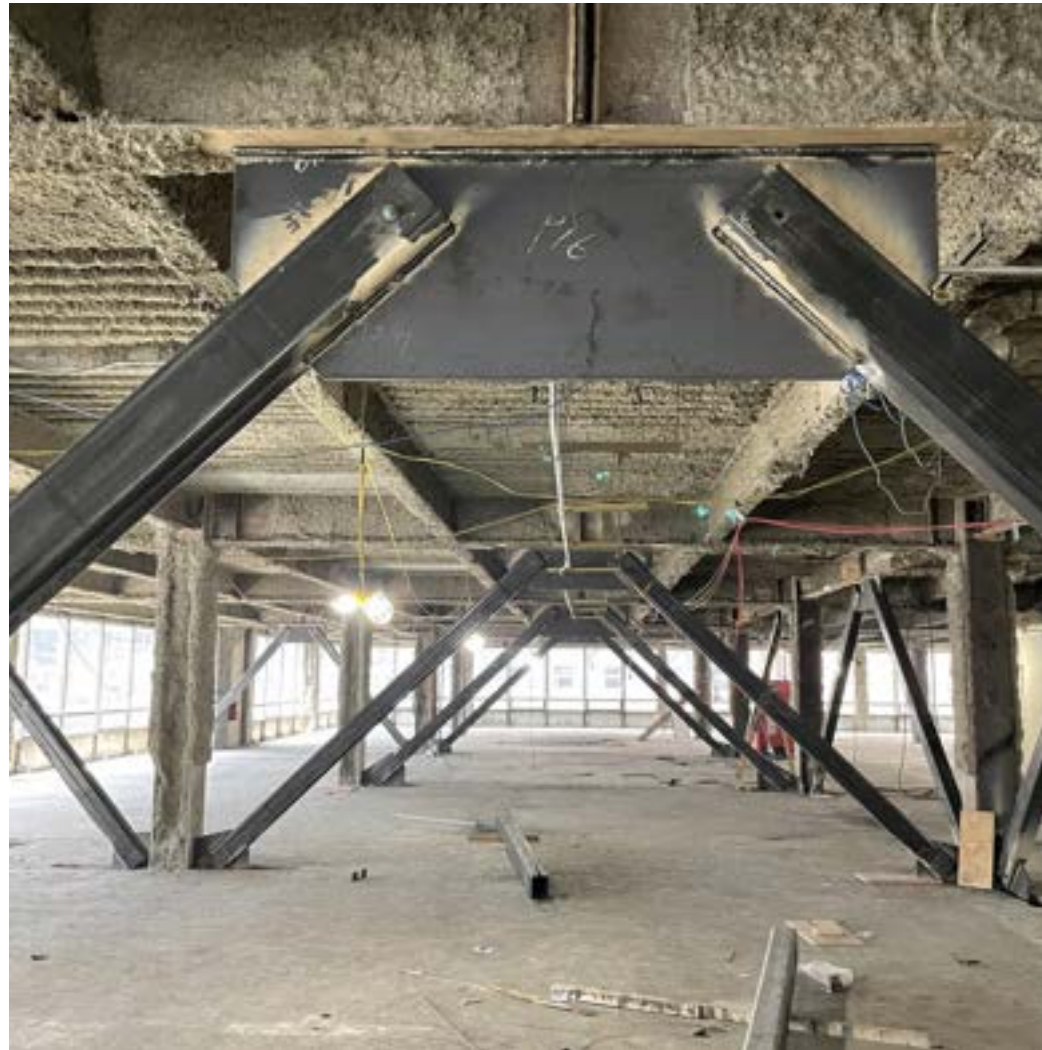
Figure 2.14. Photo of the lateral bracing being added to 160 Water.
