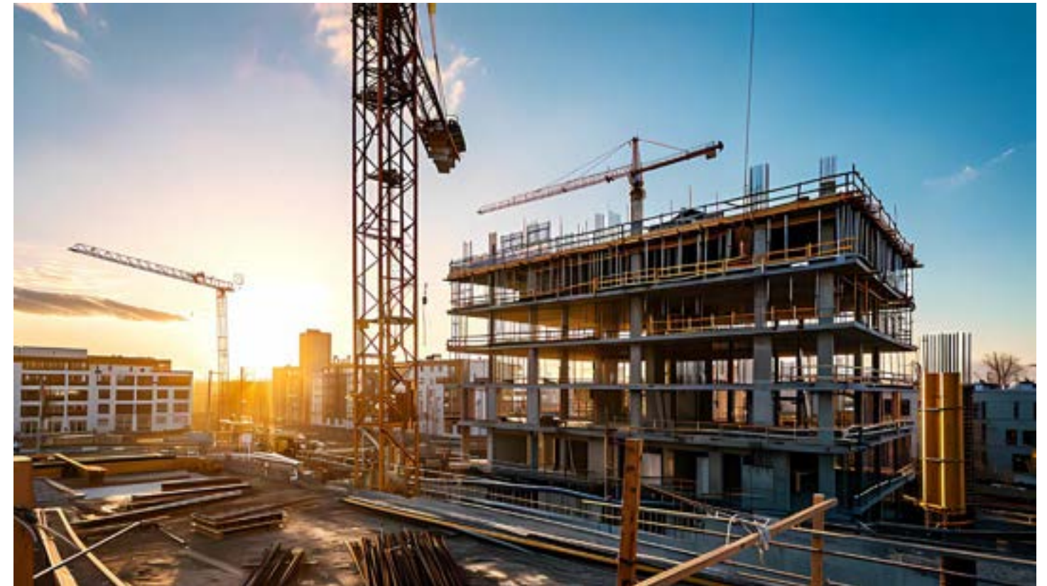
Figure 3.19. Depiction of structural steel being assembled.
