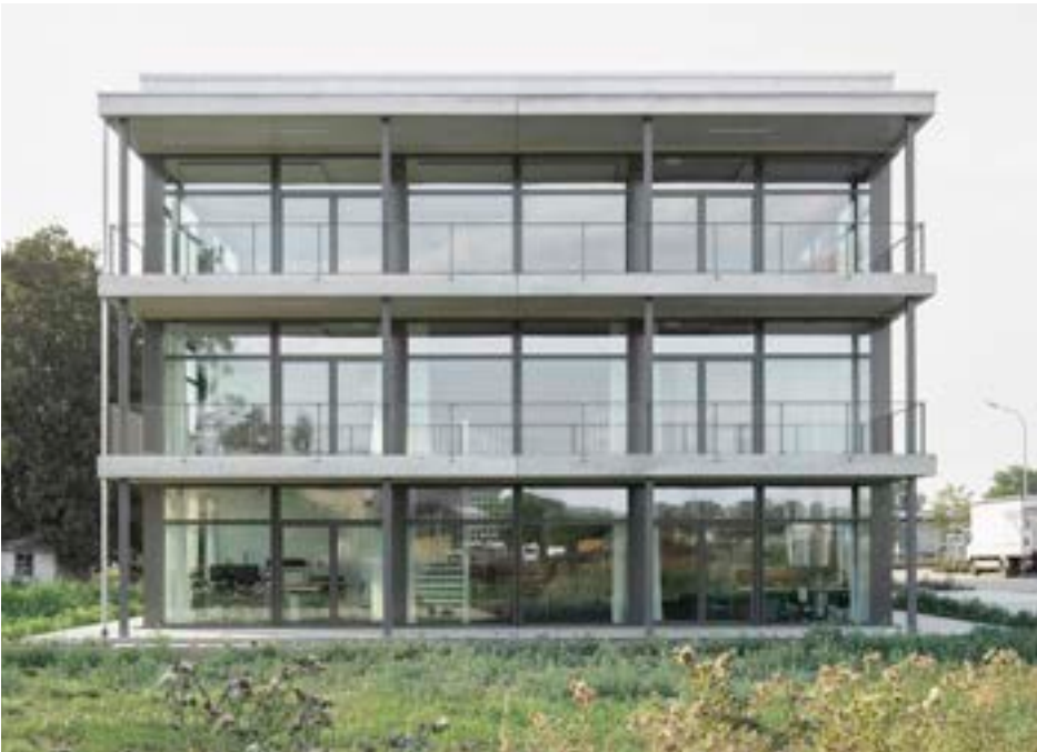
Figure 2.2. Exterior elevation of the TINA office-to-residential conversion.
