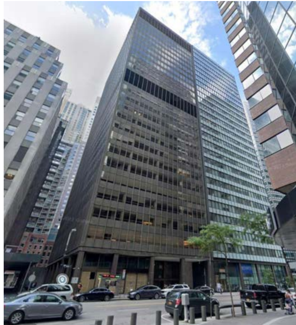
Figure 2.9. Exterior view of 160-180 Water St..
